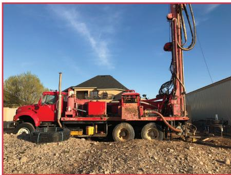
One of seven holes being drilled for the ground loop that will act as the heat exchanger between the earth and the geothermal heat pump system.
