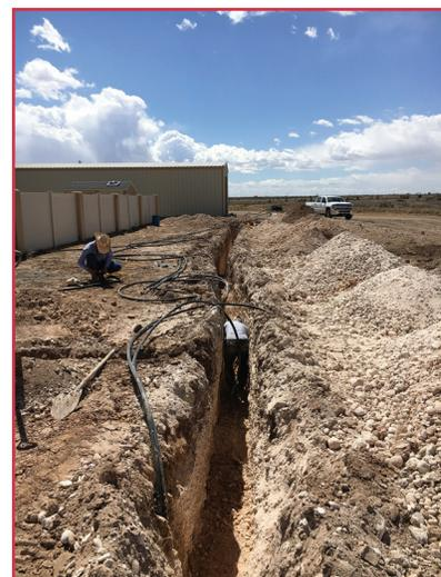
Workers preparing to connect the ground loop bore holes together.
